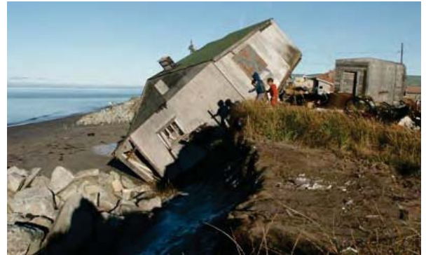
As permafrost thaws, the ground under a home in Shishmaref, Alaska collapses from erosion.
